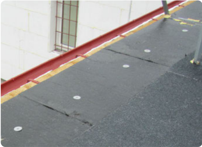
Eaves prepared for welding of top roofing felt
