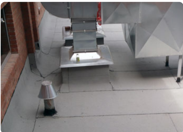
Access to ventilation equipment
