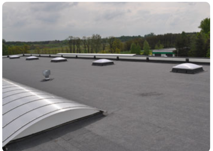
The flat roof in the system of ThermaBitum (FR)
