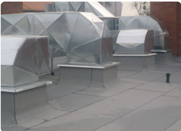
HVAC installation on a flat roof made in ThermaBitum system
