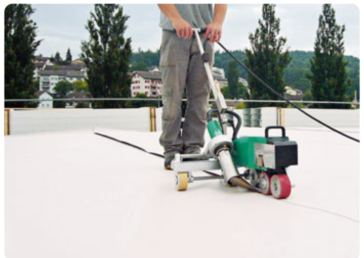
Welding longitudinal contact overlap with use of mobile, electric powered welder
