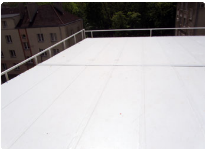
View of the roof
