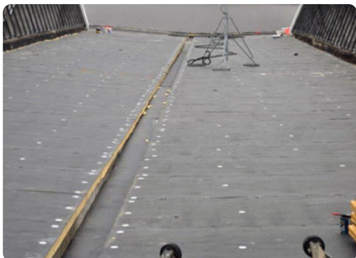
Internal gutter trough during assembly
