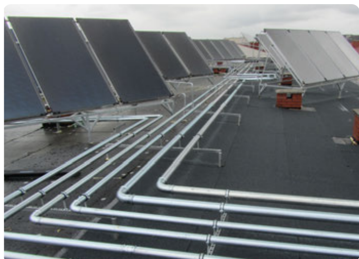
Installation of renewable energy on a flat roof insulated in the system of ThermaBitum
