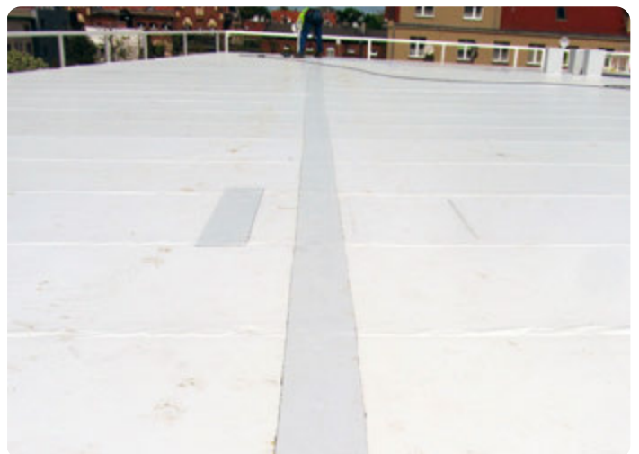
Transverse panel joint covered by welded FLAGON SV membrane strip
