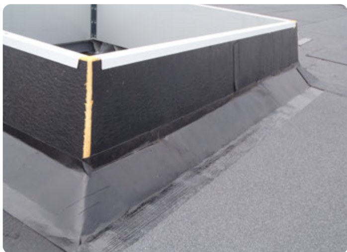
100x100 wedge at the junction with the smoke flap
