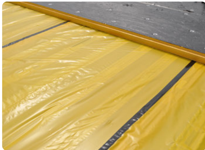
Anchoring of panels to the steel base
