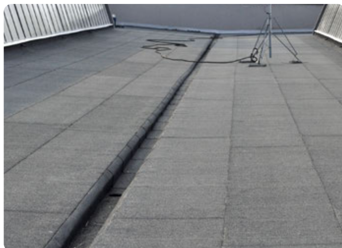
View after installation
