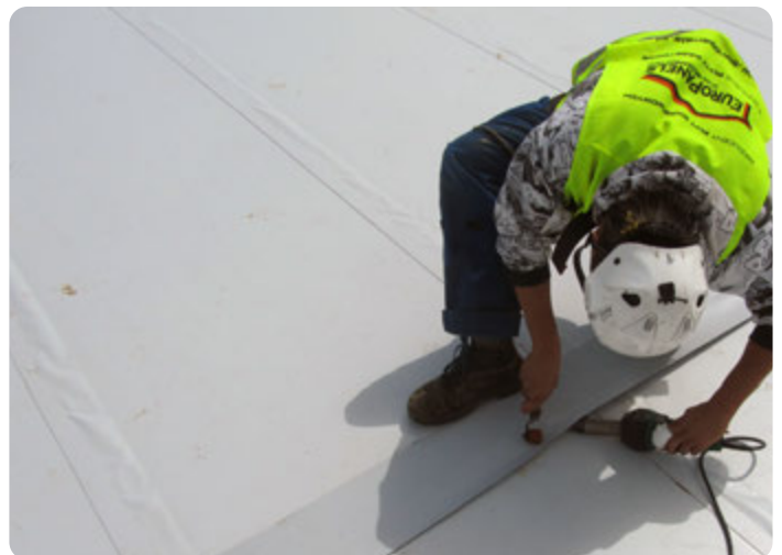
Manual welding of membrane strip on transverse panel joint
