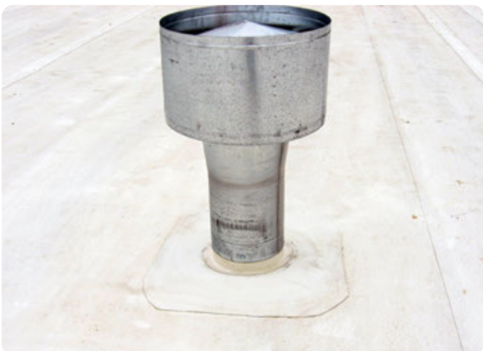
Tooling of ventilation channel
