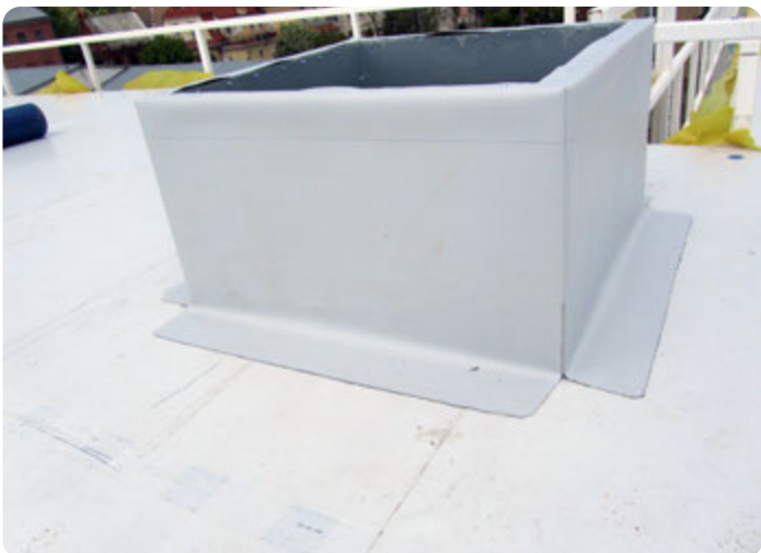
Tooling of skylight / smoke flap
