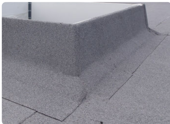
Finishing- external roofing felt
