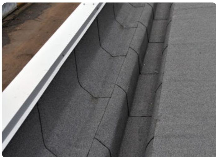
View after installation
