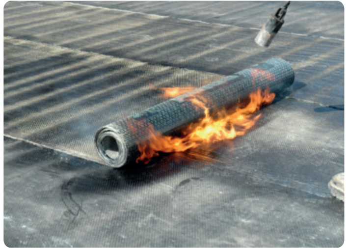
Point of welding (torch) directed to contact of felts- underlay (cladding of panels) and top (developed from a roll)
