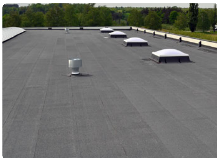
View after installation and welding of top roofing felt
