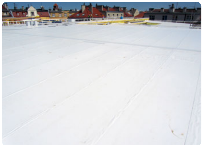
View of the roof
