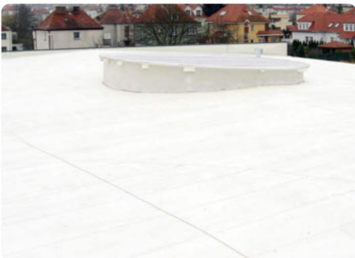
The roof after assembly
