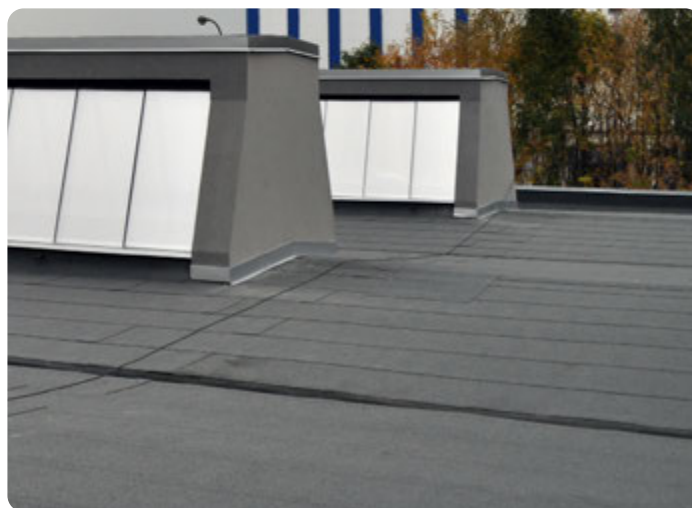
The inner gutter
