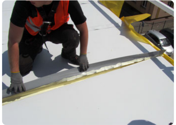
Overlap along the longitudinal panel joint
