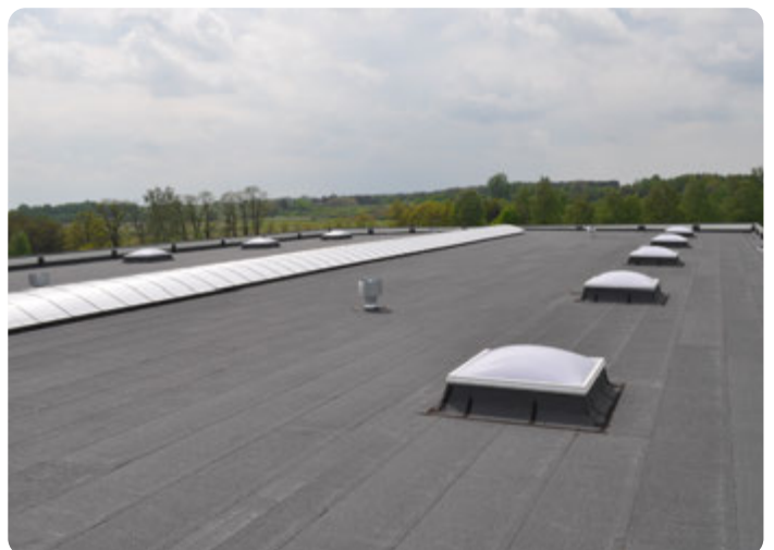
Rooftop view after the completion of ThermaBitum (FR) system
