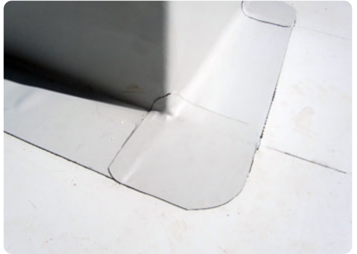
Tooling of corner
