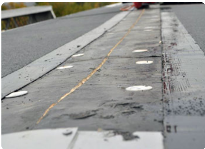
Installation in the ridge
