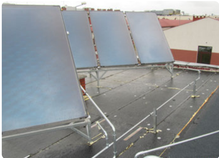
Installation of renewable energy systems
