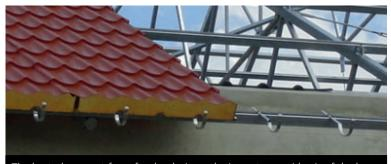
The best placement for rafter hooks is on the inner trapezoid axis of the lower <u>cladding.</u> Montage in every second trapeze gives a spacing of 530mm.
