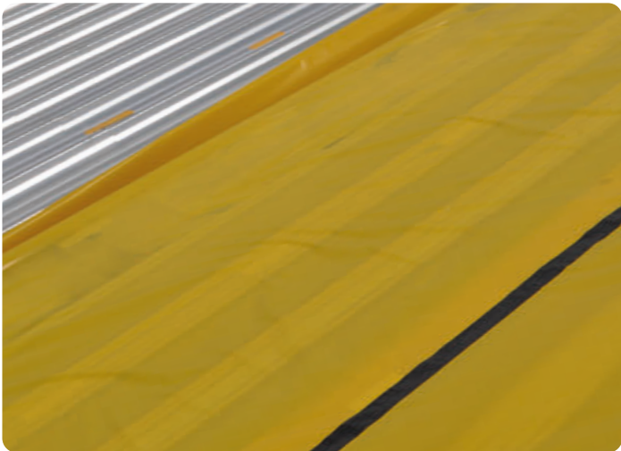
Preparation for installation: a vapor barrier on steel base
