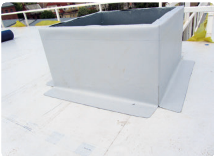
Tooling of skylight / smoke flap
