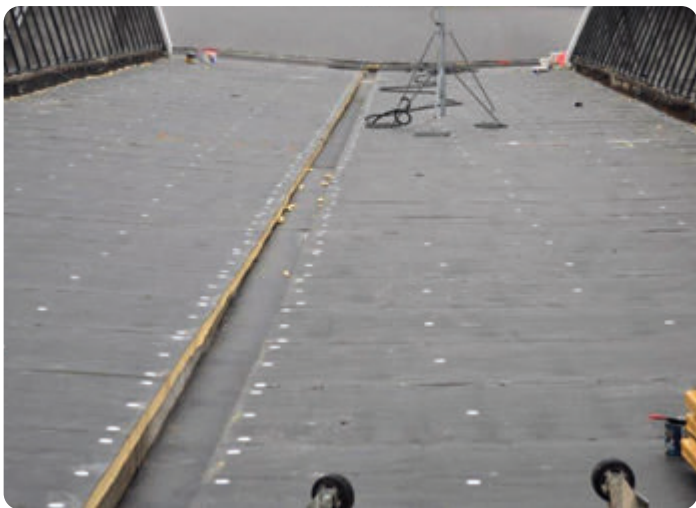
Internal gutter trough during assembly
