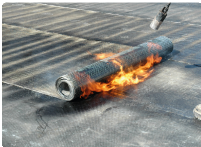
Point of welding (torch) directed to contact of felts- underlay (cladding of panels) and top (developed from a roll)
