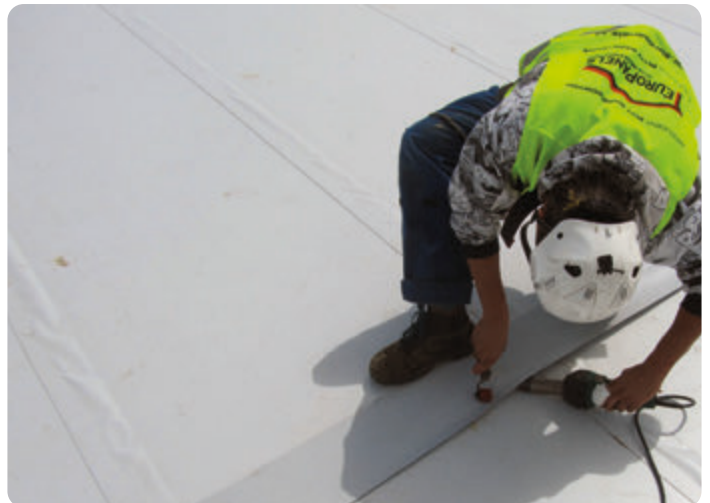
Manual welding of PVC membrane strip on transverse panel joint
