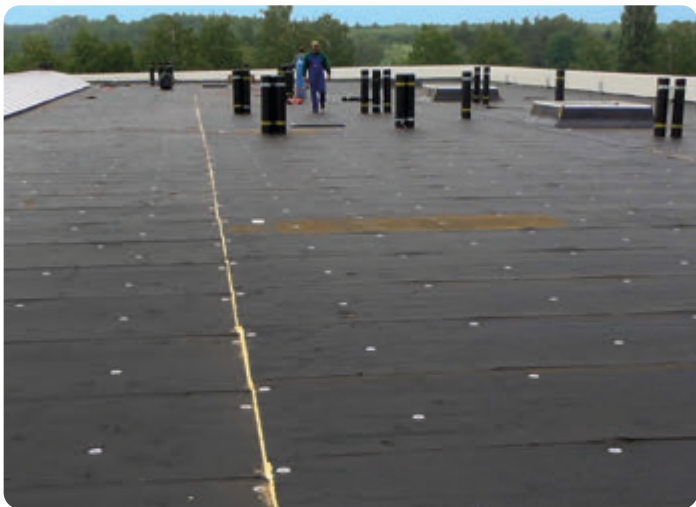
Mounting of ThermaBitum panels on the roof
