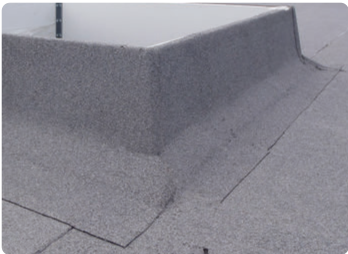
Finishing- external roofing felt
