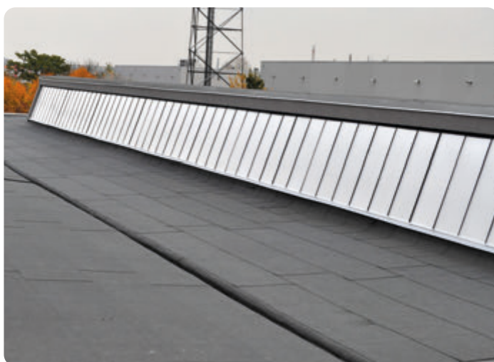
Internal gutter and skylights in the system of ThermaBitum
