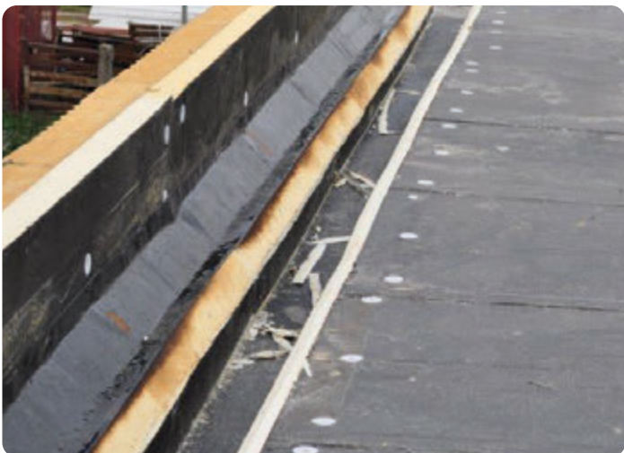
Gable wall insulation (firewall) with an internal gutter trough
